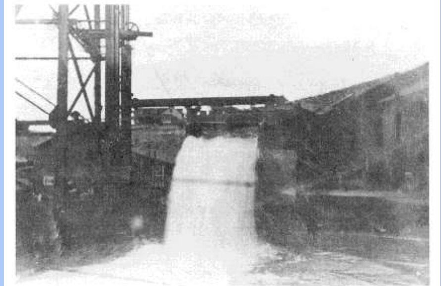
Water discharge from the Boom Shaft; 4,000,000 gallons per day, 1908. Macia-Devere Collection
